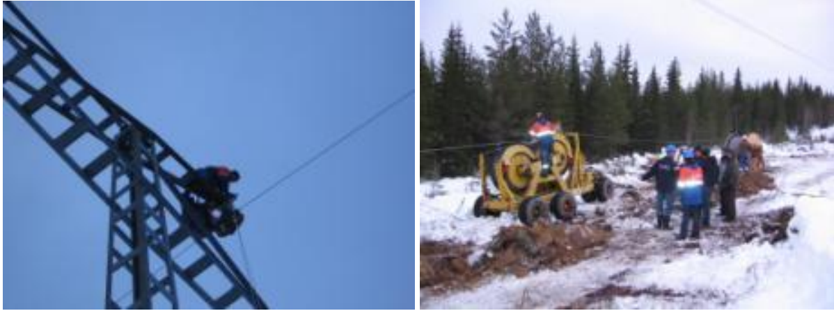
Figure 4 Laying out the ground wire on the pulley blocks (left) and work place with puller and cable drum battery – works executed in Sweden (picture by B.Dudek)
